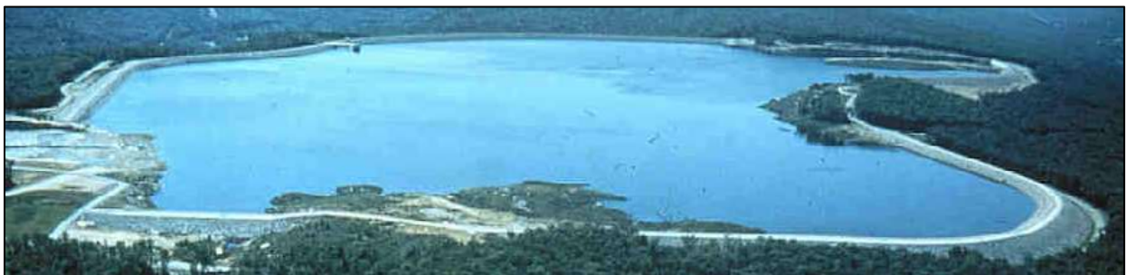
Figure NFM-AIR#6-2. Northfield Mountain Upper Reservoir Aerial Photo
