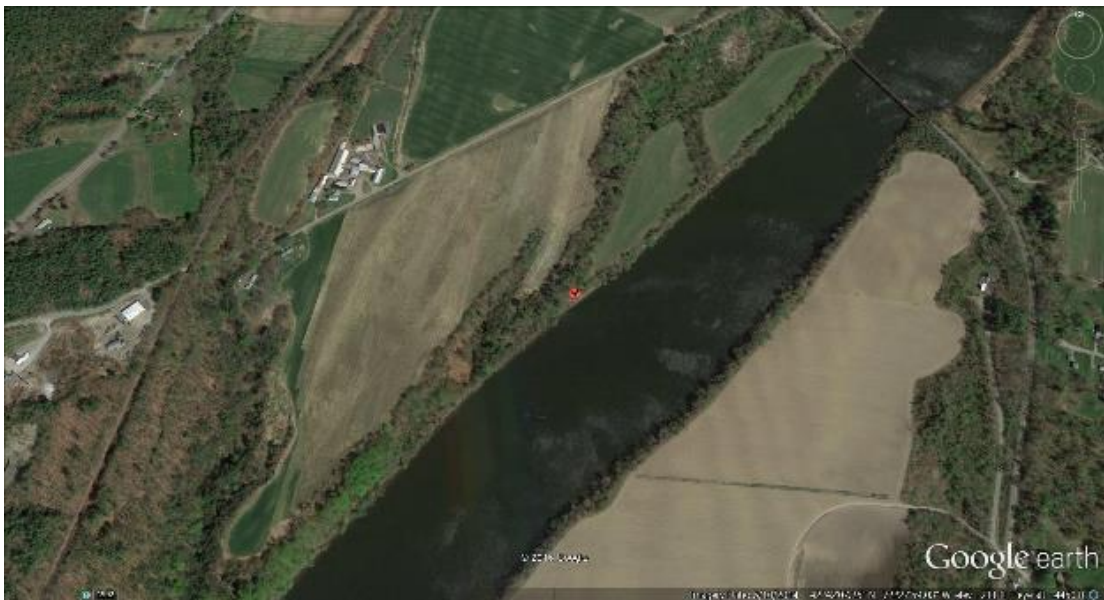
Figure 5.5.4-5: Irrigation pumping from the Connecticut River and Location on Google Earth, Photo 255
