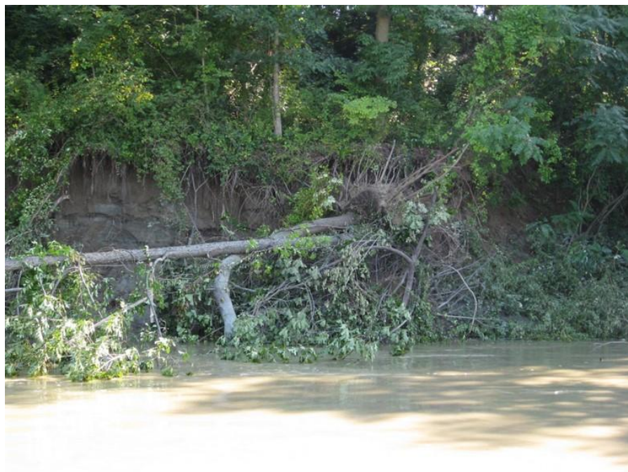
Figure 5.5.5.5-17 Erosion Due to High Flow in 2011
