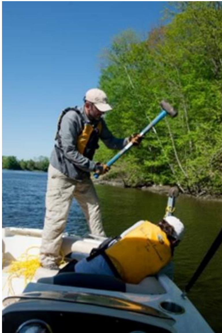
Figure 4.2.8.2-9: Installation of the T-posts
