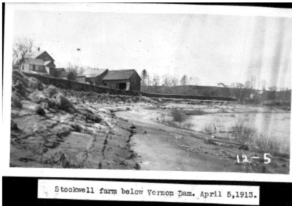
Figure 5.5.5-5 Eroded Bank in Turners Falls Impoundment Downstream of Vernon Dam – April 5, 1913 (TransCanada)
