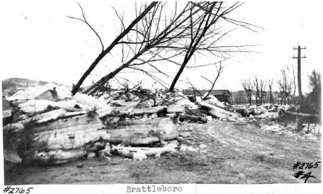
Figure 5.5.5.2-3 Ice along riverbanks showing damage to trees, 1915 (after TransCanada)
