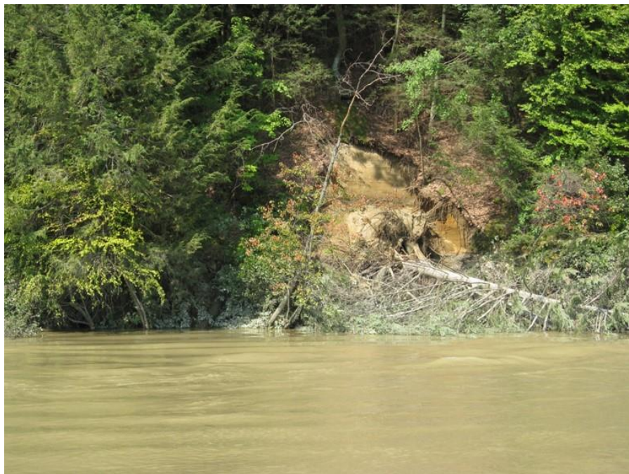
Figure 5.5.5.5-16 Erosion Due to High Flow in 2011
