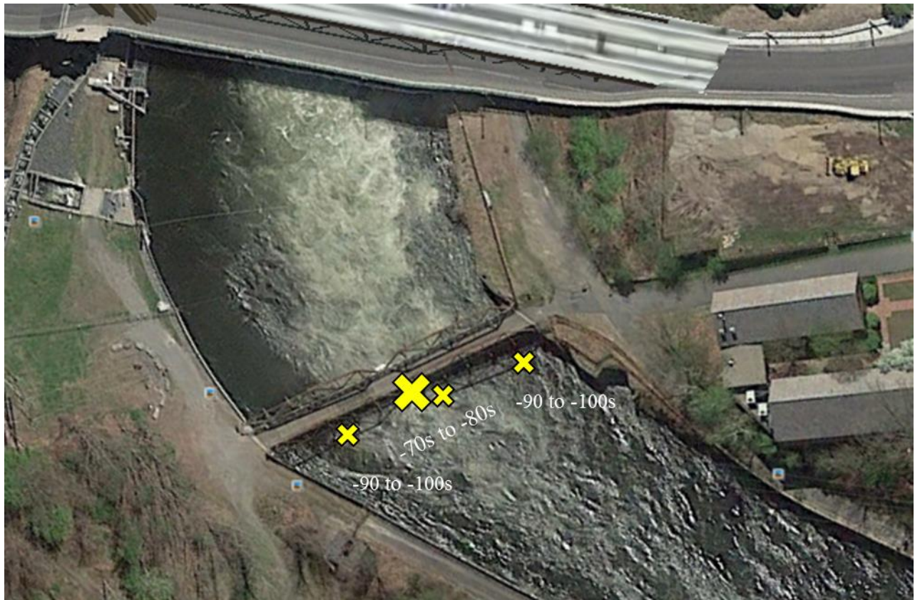
Figure A-10: The large X marks the approximate placement of the Yagi antenna used, in conjunction with an Orion receiver, to detect fish moving through the power canal downstream of the Gatehouse. Small X's mark the approximate placement of three in-water droppers used at this location to assist with monitoring the passage of downstream eel. The radio tag was tested at a depth of approximately 2 to 3 ft. Power levels remained consistent around -70 to -80 dB across the canal, and attenuated out to -90 dB downstream of the bridge.
