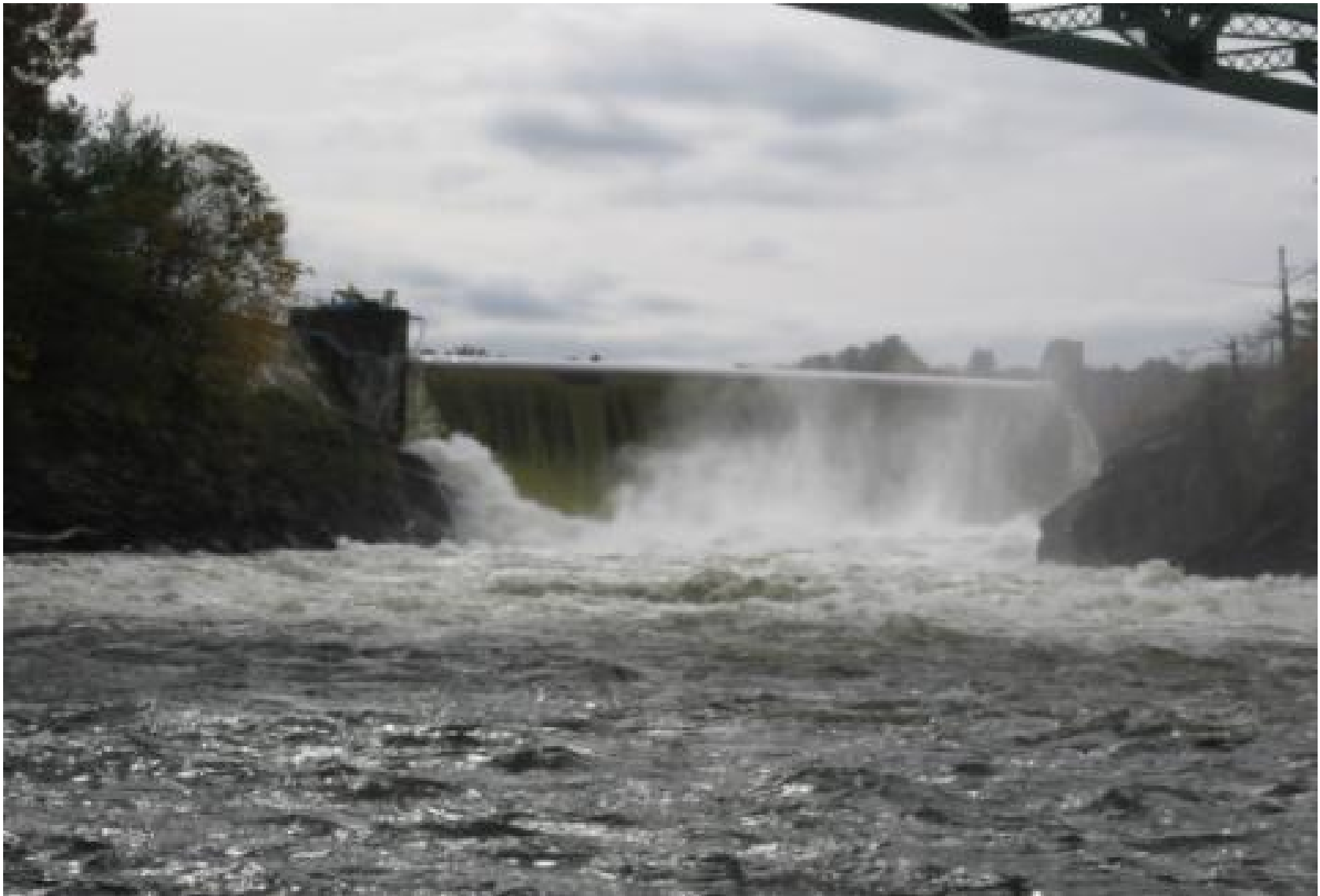
Figure 2-3: Downstream of Bascule Gate 4.
