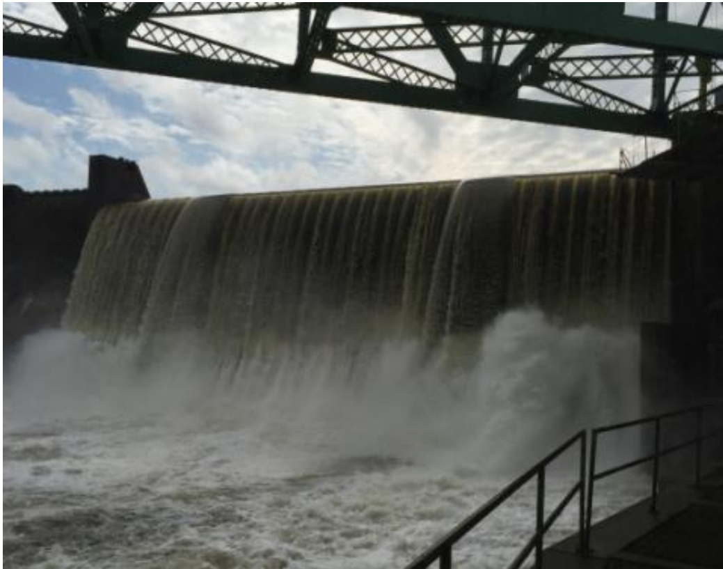
Figure 2-2: Downstream of Bascule Gate 1.
