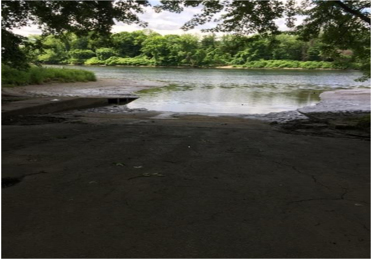
Pauchaug Boat Launch – showing narrow channel cut and accumulated sediment on both sides of boat launch. Turners Falls Impoundment elevation at the time of this picture was 180.3 ft.
