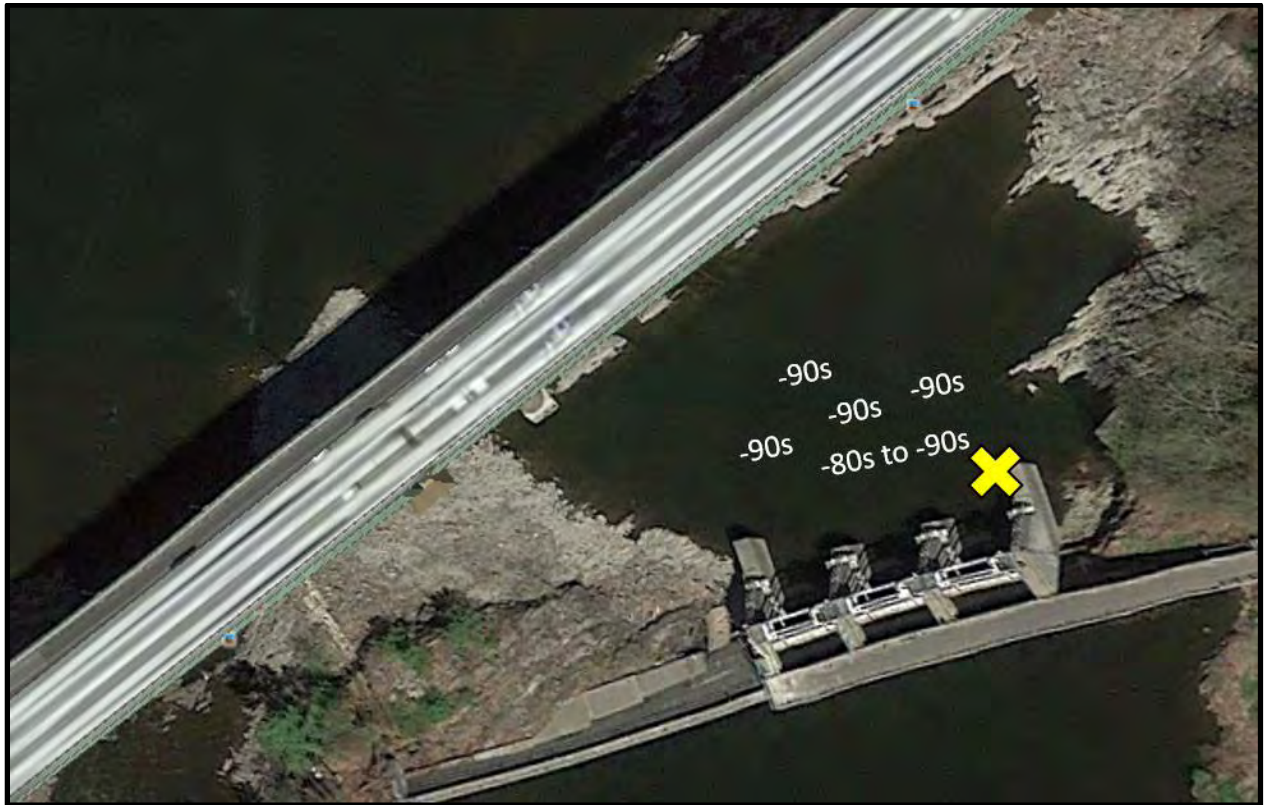
Figure 12: The large yellow X marks the approximate placement of the yagi antenna and the Orion receiver used to detect fish below Turners Falls Dam at River Mile 122. The radio test tag produced power levels ranging from -80 to -90s with highest powers located closest to the yagi antennas and attenuated farther out from the antenna.
