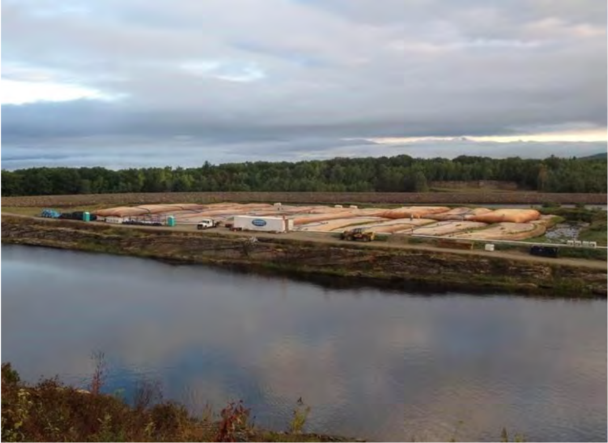
Figure 2.4-3 Geotube Dewatering System
