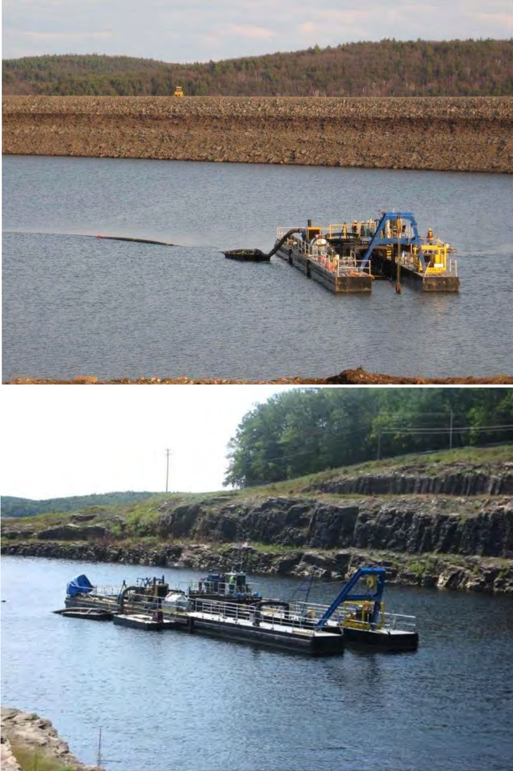
Figure 2.4-2 Dredge Equipment Setup
