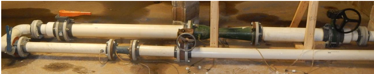
Figure 4-15: Venturi type flow meters for measuring river flow.
