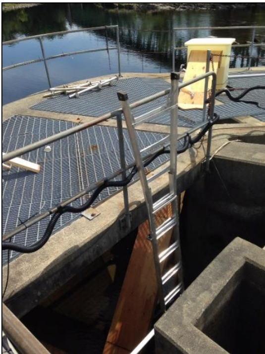
Spillway Fishway eel trap, located within the second turning pool
