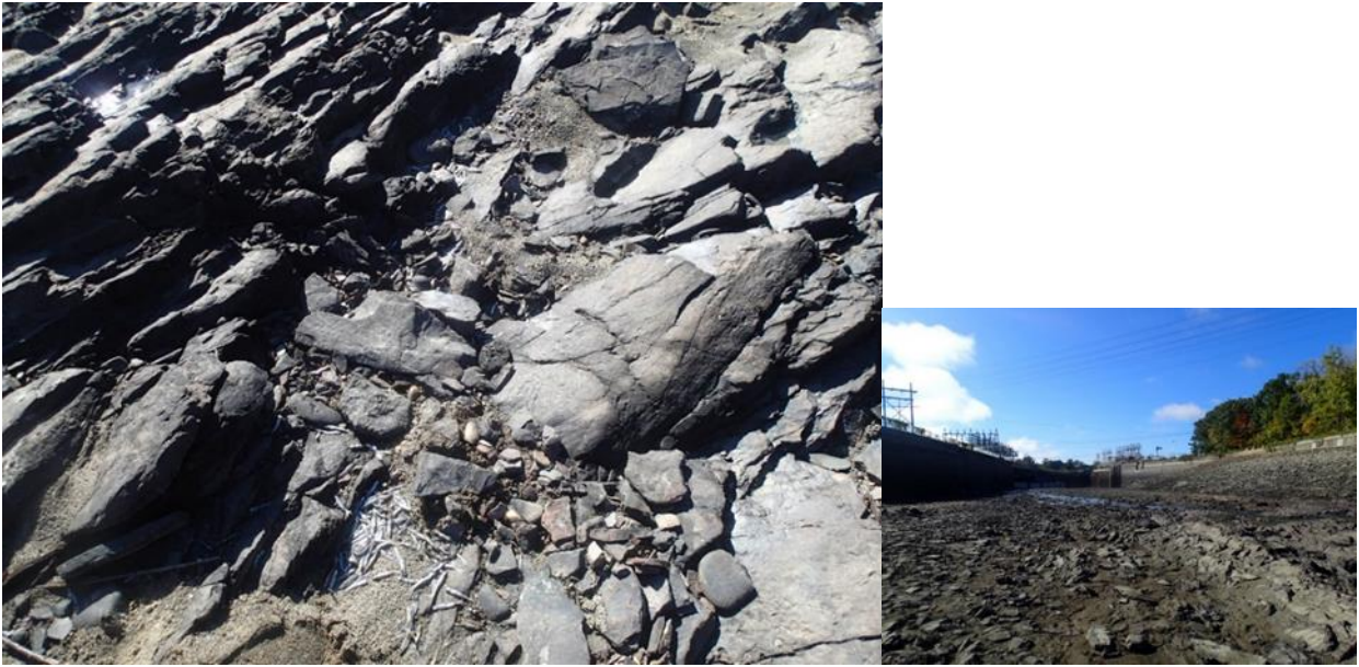
Figure 3.1-8. Stranded Fish among Bedrock, located Upstream of Cabot station, near Wall to river left
