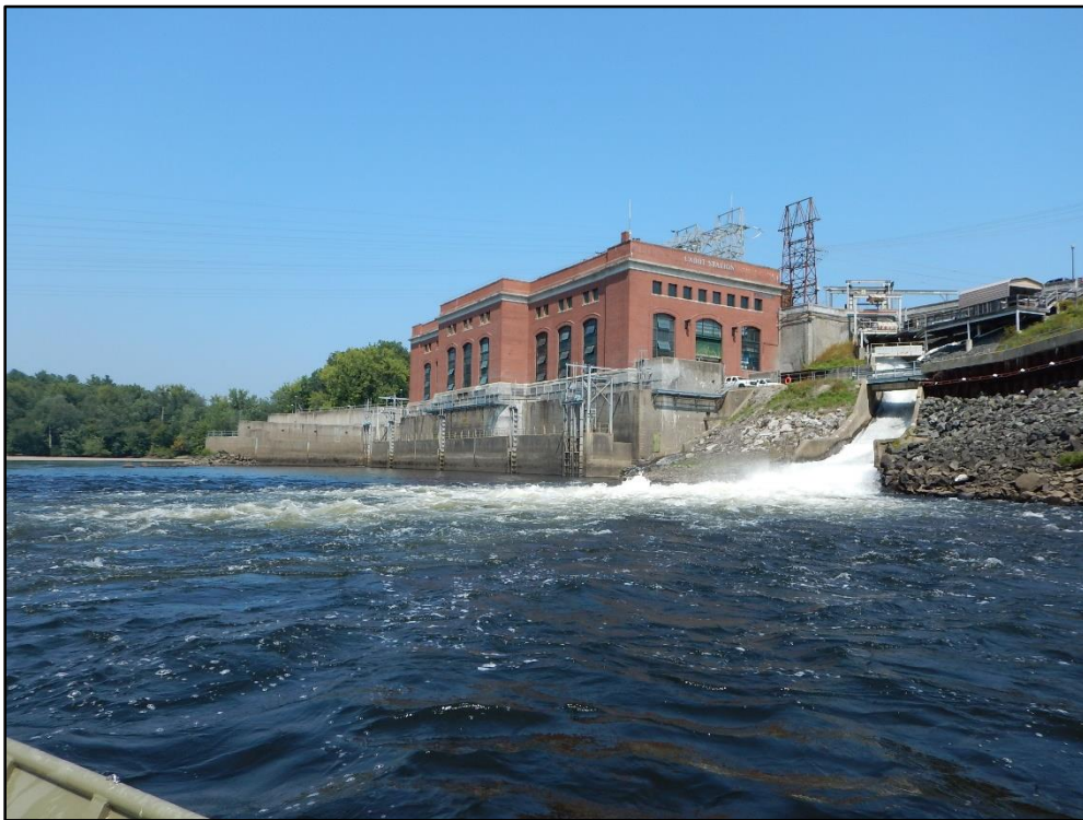
Upstream View of Sluice Gate discharge location
