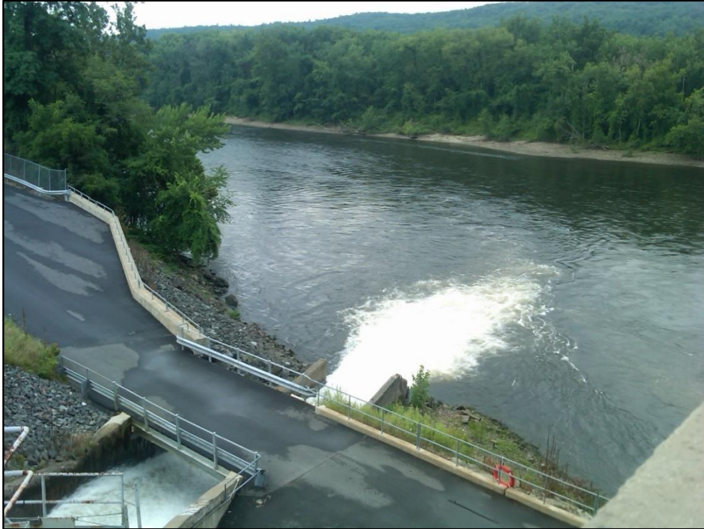
View of Sluice Gate discharge during typical operation, from above
