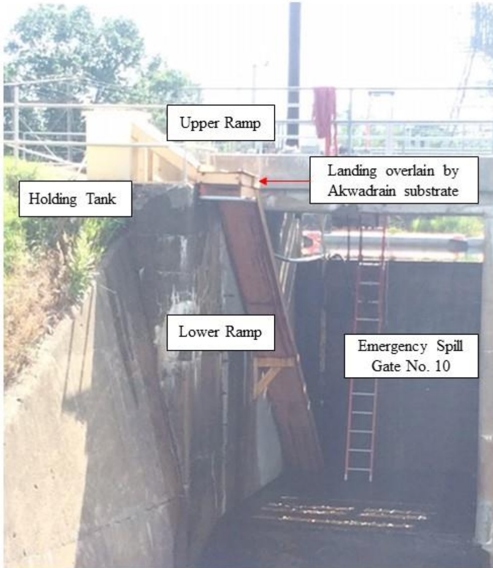
Figure 3.0-4: The Temporary Eel Trap Located at Gate No. 10 of the Cabot Emergency Spillway at the Project, Turners Falls, MA
