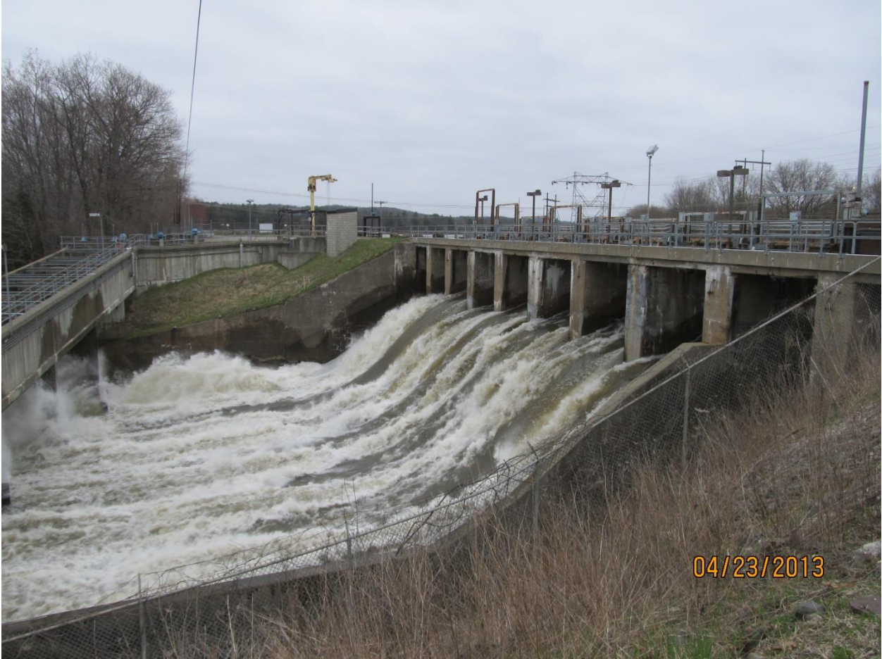
Figure 5.0-1: Cabot Emergency Spillway, Turners Falls, MA
