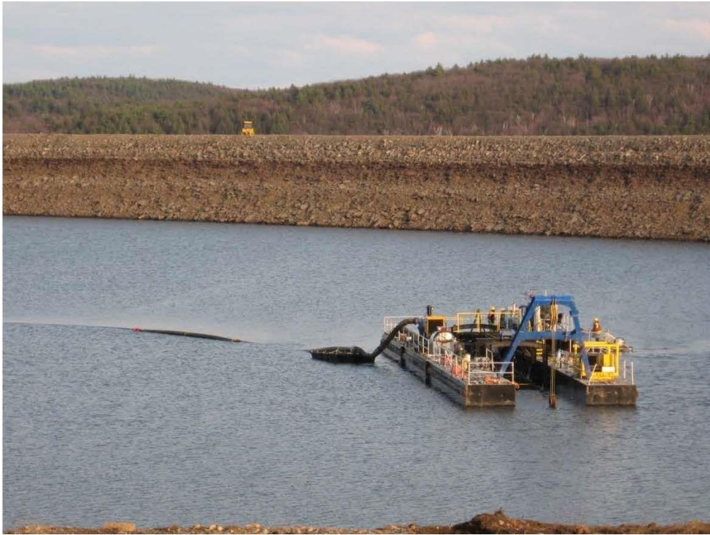
Figure 2.4-2 Dredge Equipment Setup
