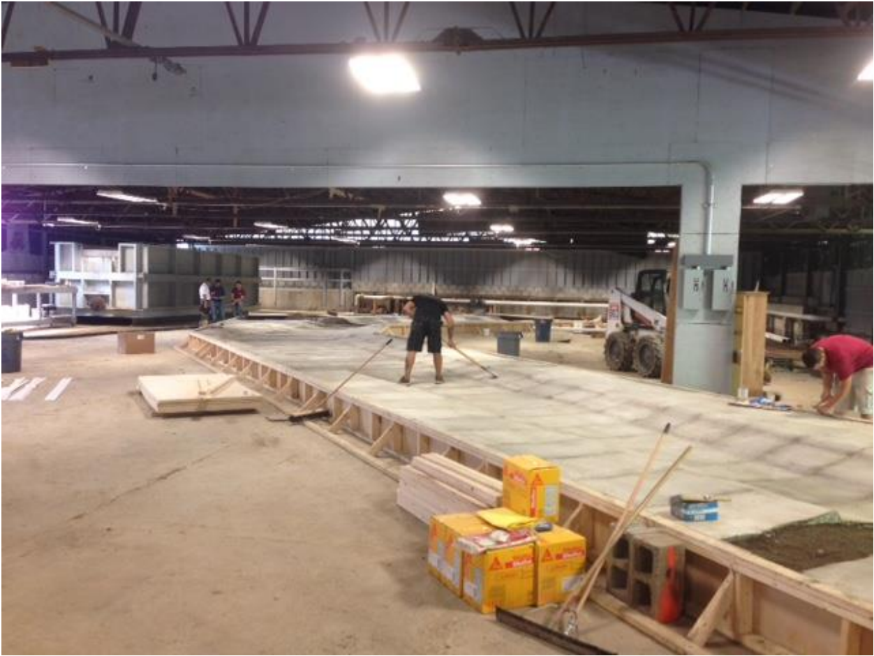
Figure 2.3.3-4 Physical Model of Northfield Tailrace Area- Looking Downstream toward Tailrace
