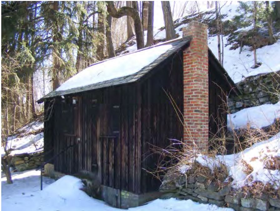
2014 View of Restrooms (Source: TRC)
