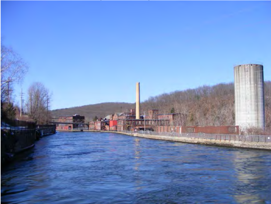
2014 View of Power Canal and Keith's Mill Footbridge
