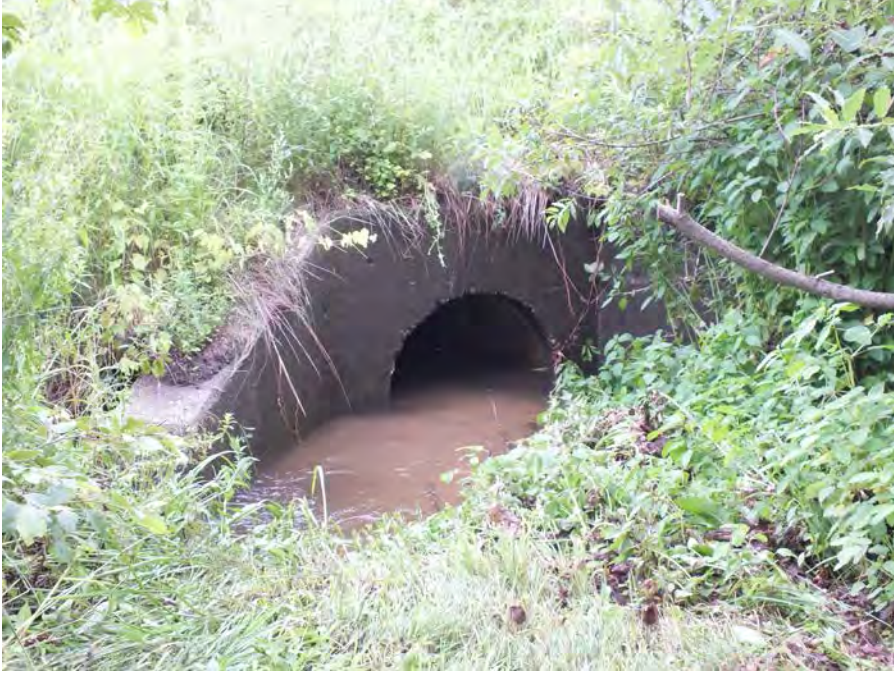
2015 Photo of Culvert at Chappell Drive (Source: TRC)
