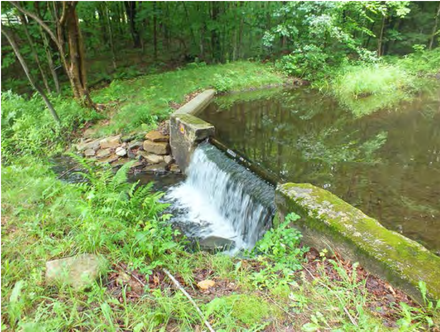
2015 View of Dam (Source: TRC)
