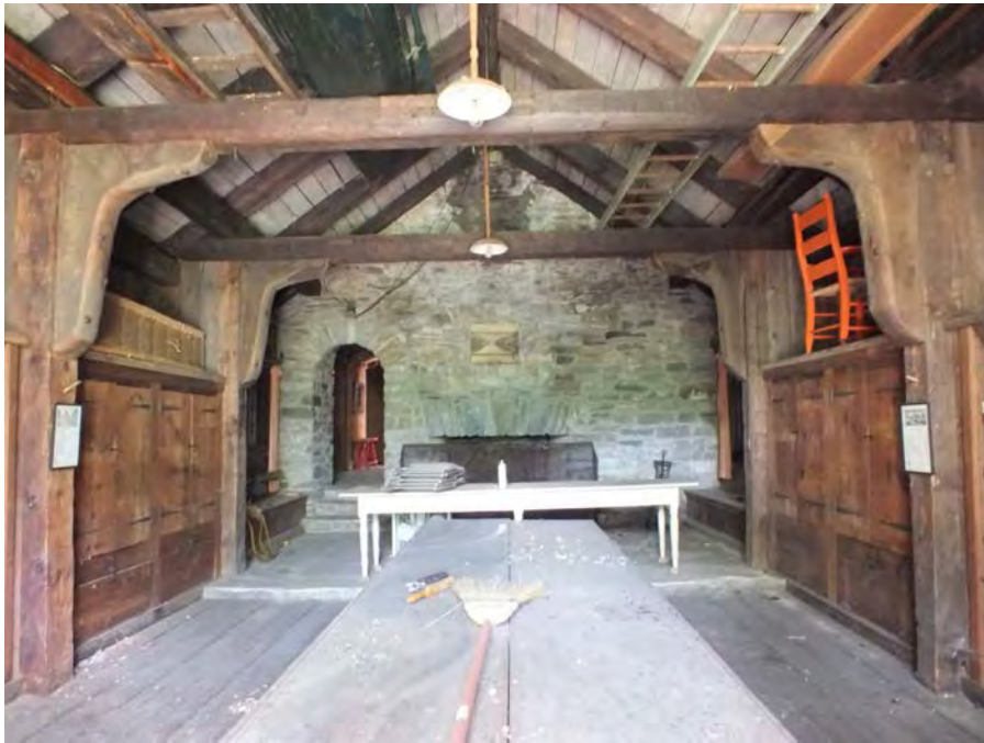
2015 Interior View of Western Section (Source: TRC)
