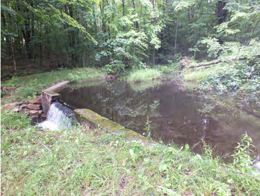
2015 View of Dam (Source: TRC)
