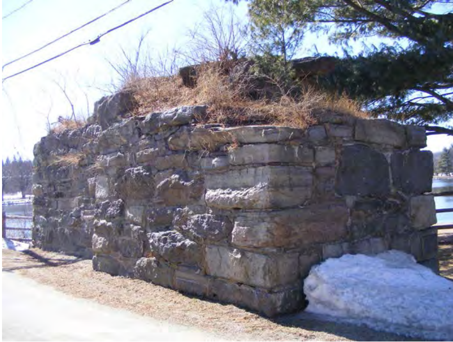
2014 View of Extant Abutment in Gill (Source: TRC).
