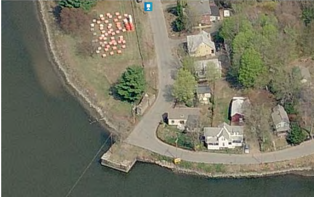
2008 Low-level oblique image of Red Suspension Bridge Abutment (Source: MASSDOT GIS)
