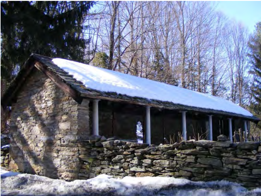
2014 View of East and South Elevations of Carriage House (Source: TRC)
