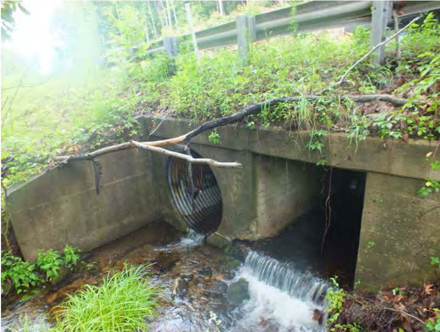
2015 Photo of Culvert at Packard Brook (Source: TRC)
