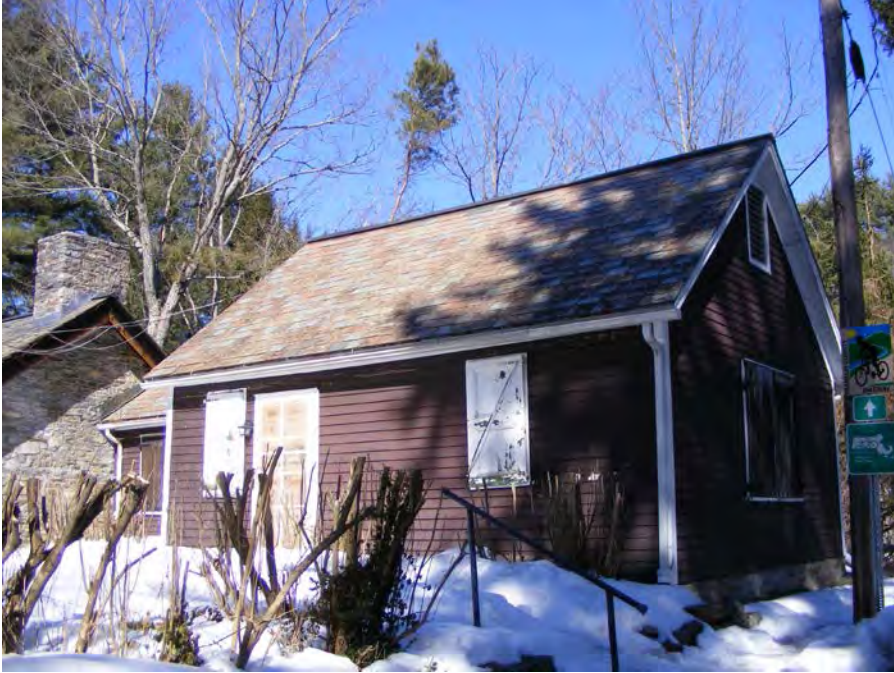
2014 View of Eastern Section (Source: TRC)
