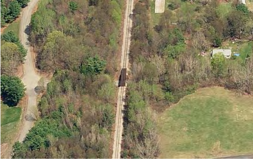
2008 Low-level oblique image of Central Vermont Railroad Bridge (Source: MASSDOT GIS)
