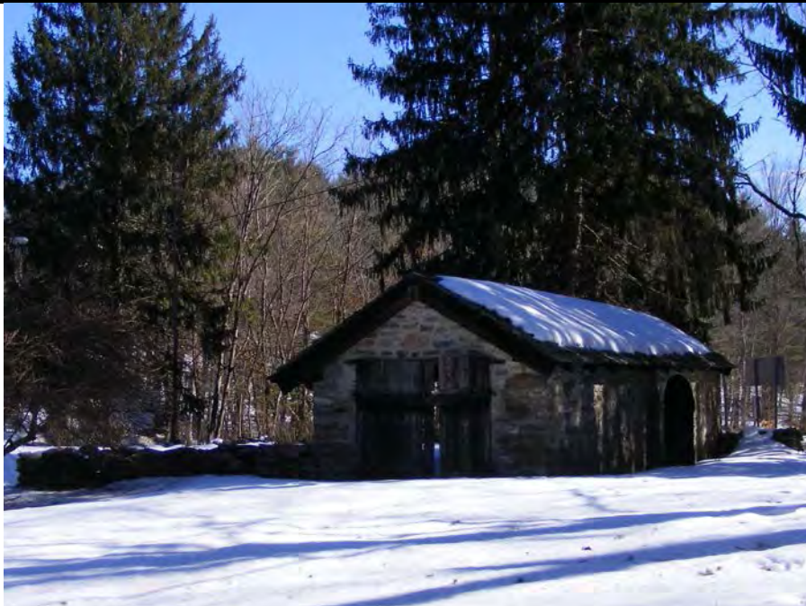
2014 View of North and West Elevations of Carriage House (Source: TRC)
