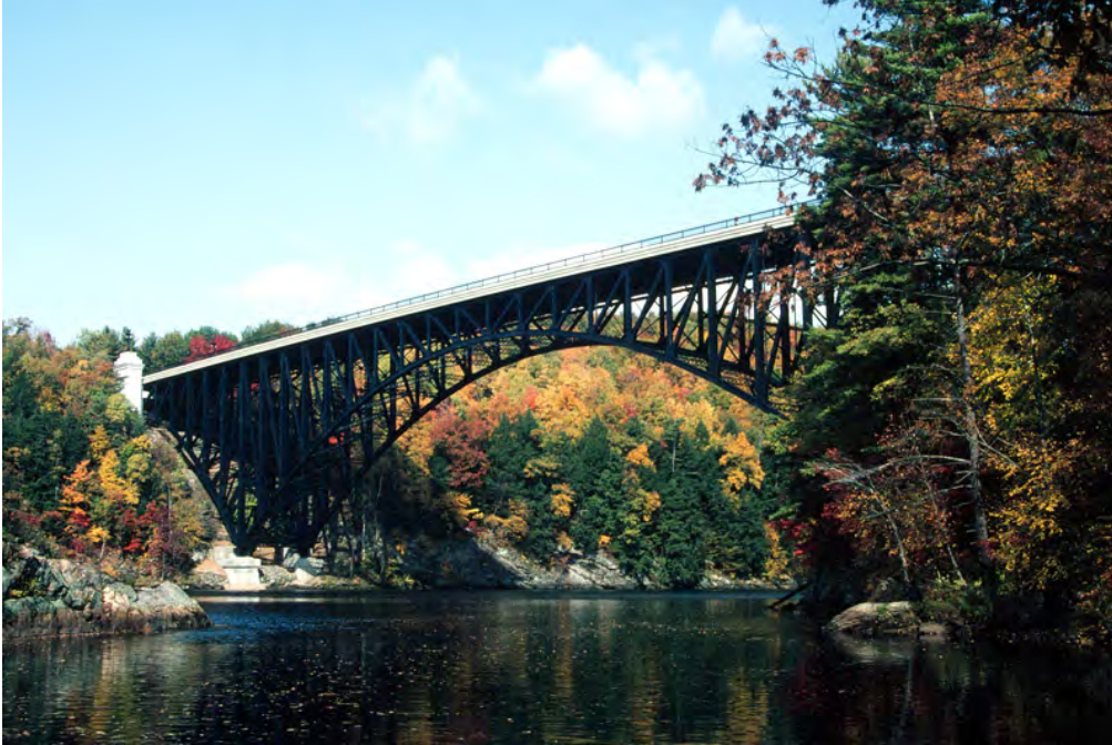
French King Bridge along Mohawk Trail (Source: MassDOT)
