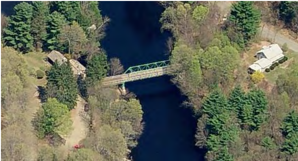
2008 Low-level oblique image of French King Bridge over Connecticut River (Source: MASSDOT GIS)
