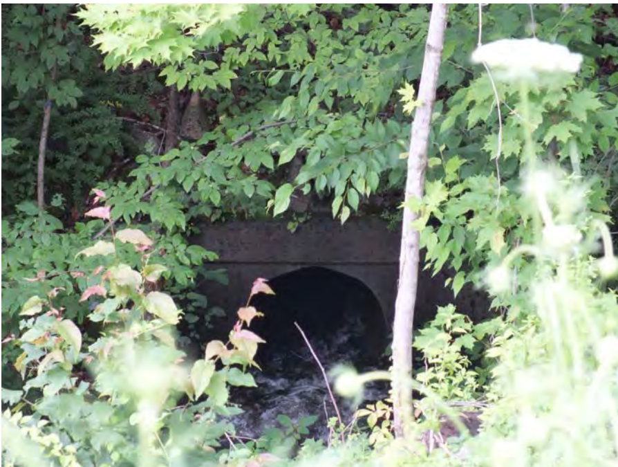
2015 Photo of Culvert at Pisgah Mountain Road (Source: TRC)
