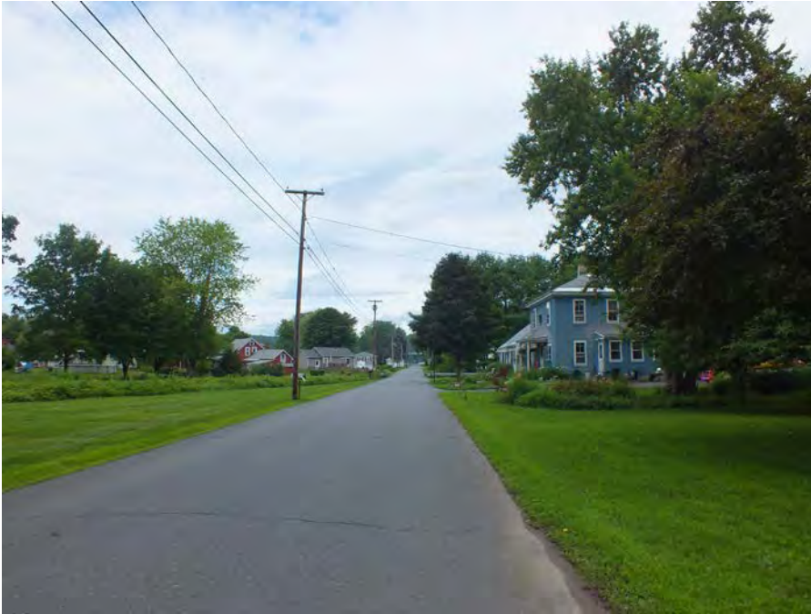
Streetscape along Oak Street (Source: TRC 2015)
