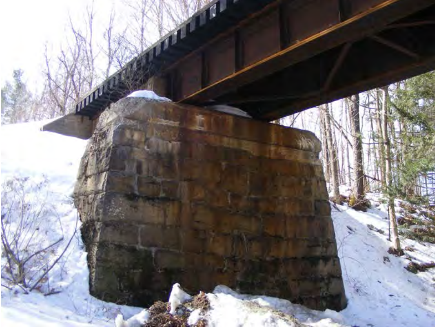
2014 View of South Abutment (Source: TRC)
