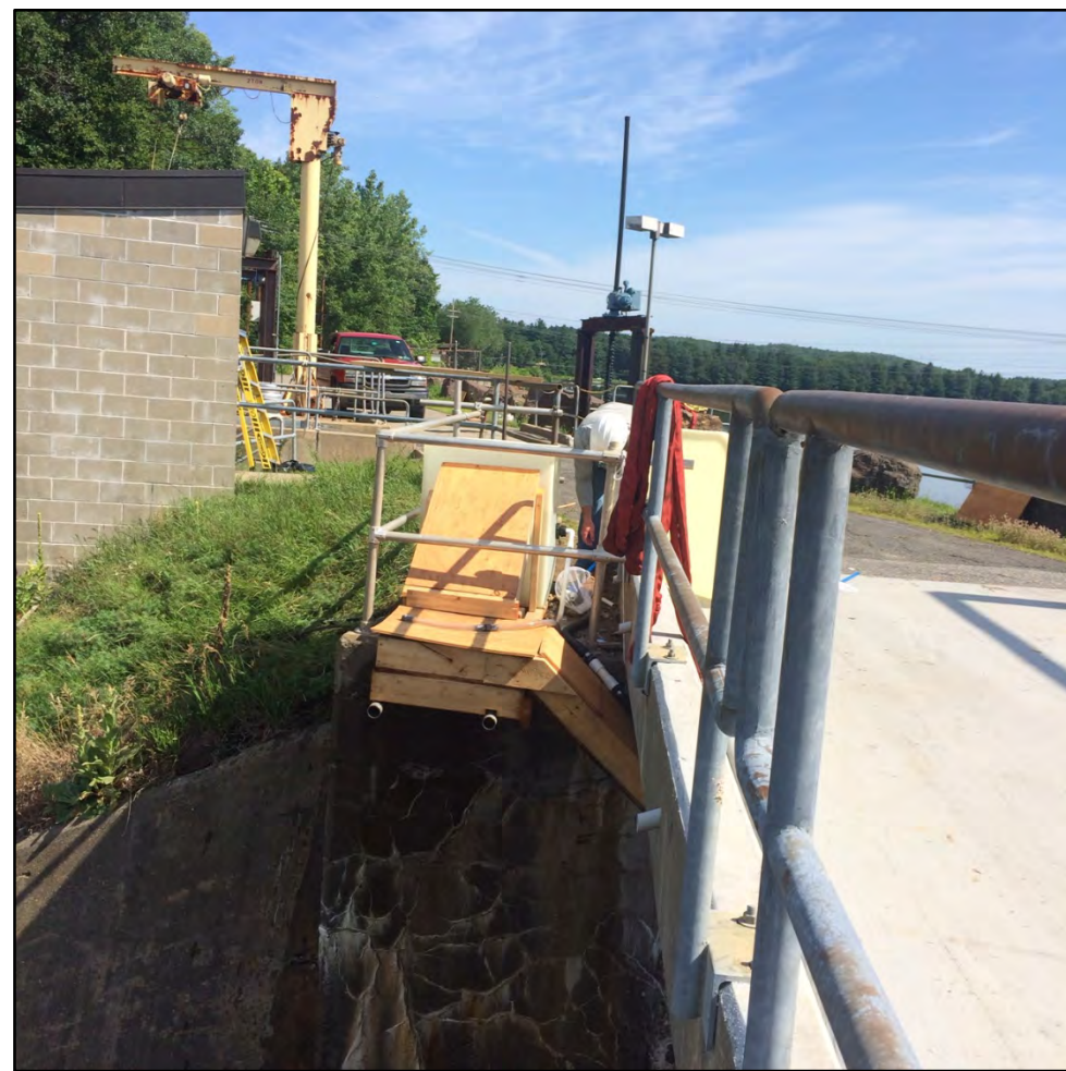
Cabot Emergency Spillway Eel Ramp
