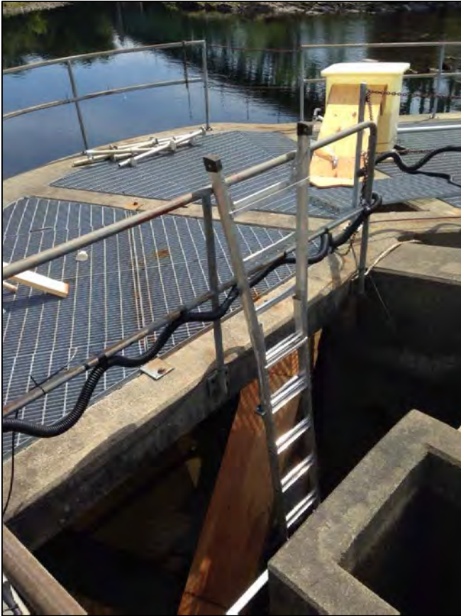
Spillway Ladder Trap
