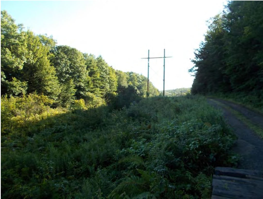
Figure 4.2.7-1. Representative view of the right-of-way community.
