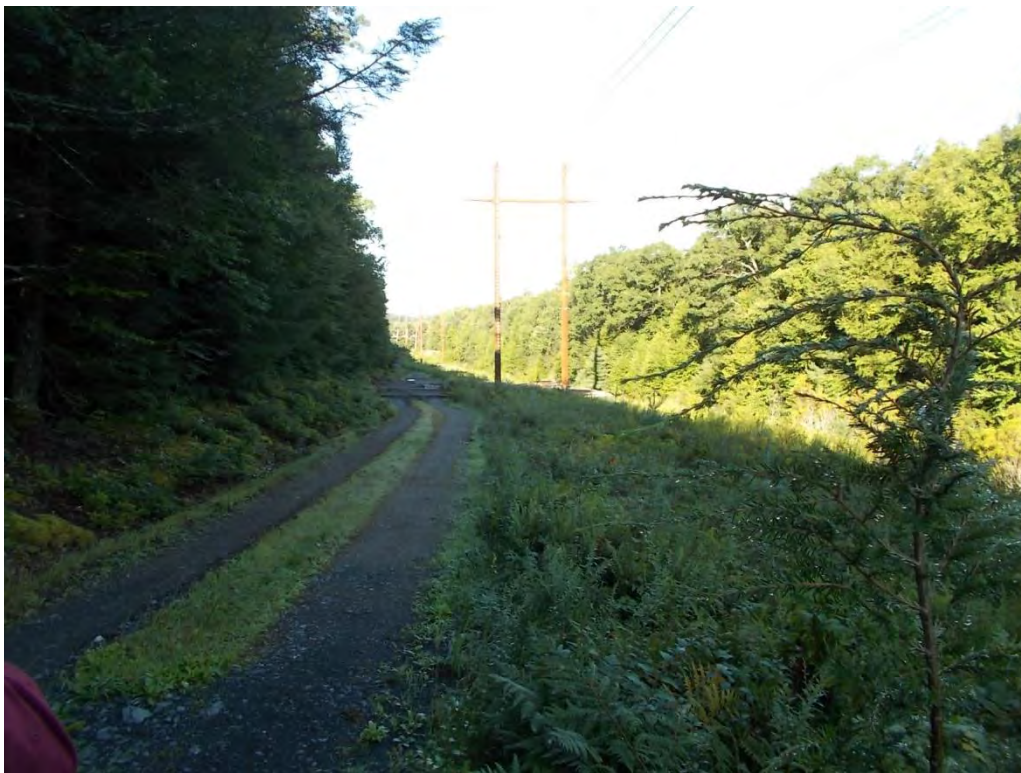
Figure 4.4-3: Example of Habitat Along Eversource Transmission Right-of-Way
