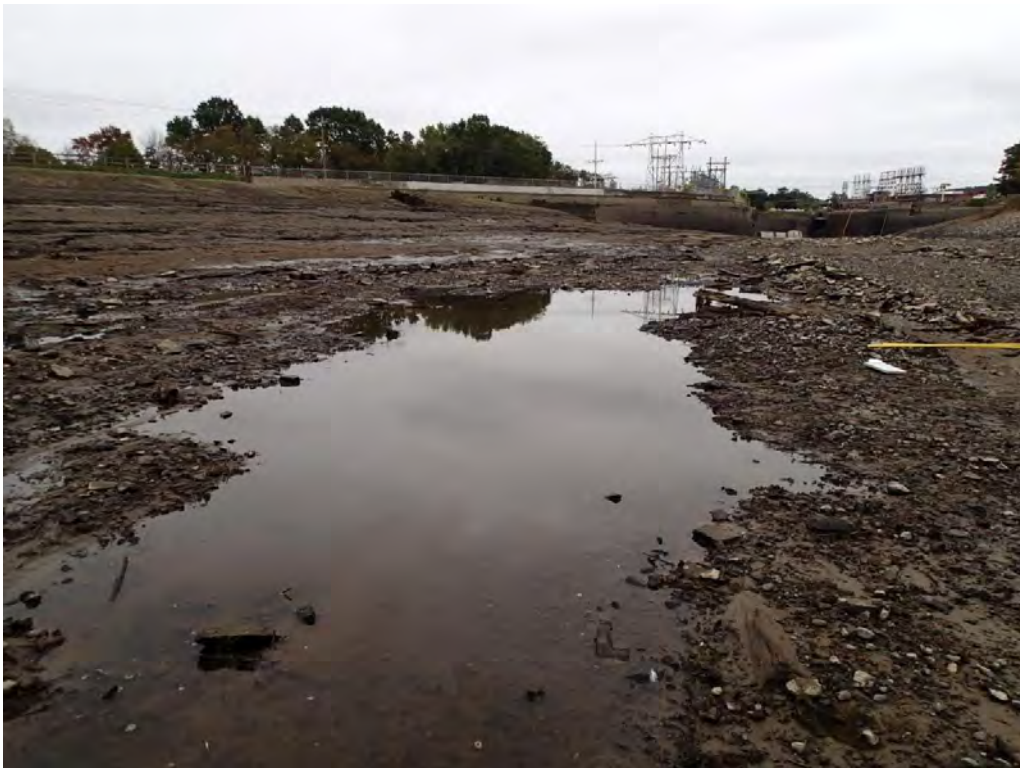
Photo 4. View from center of Zone 2 looking downstream towards powerhouse (Day 1).
