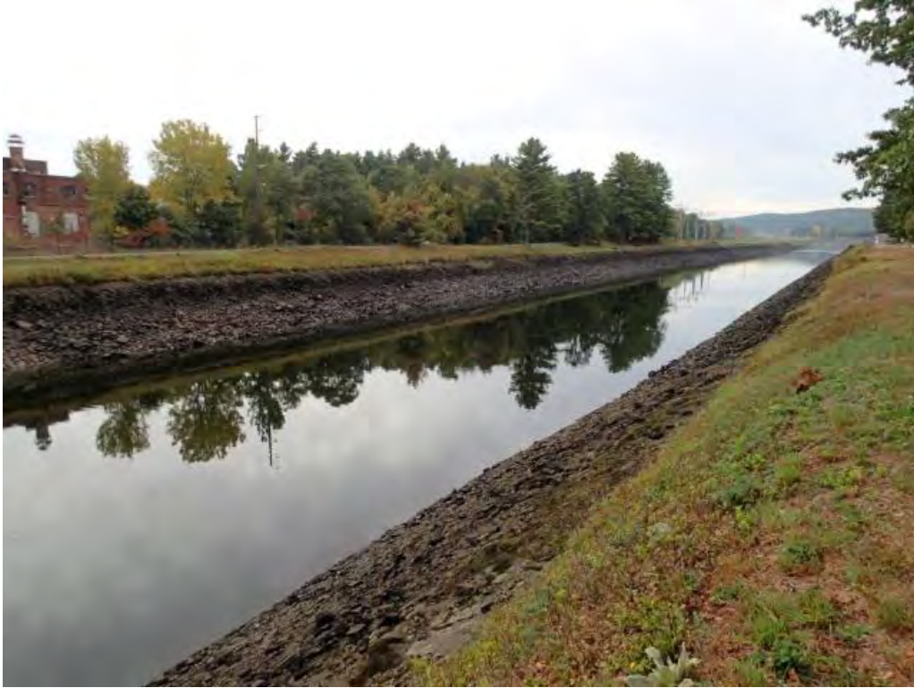
Photo 11. Typical condition of upper, narrow portion of canal during drawdown (Day 1).
