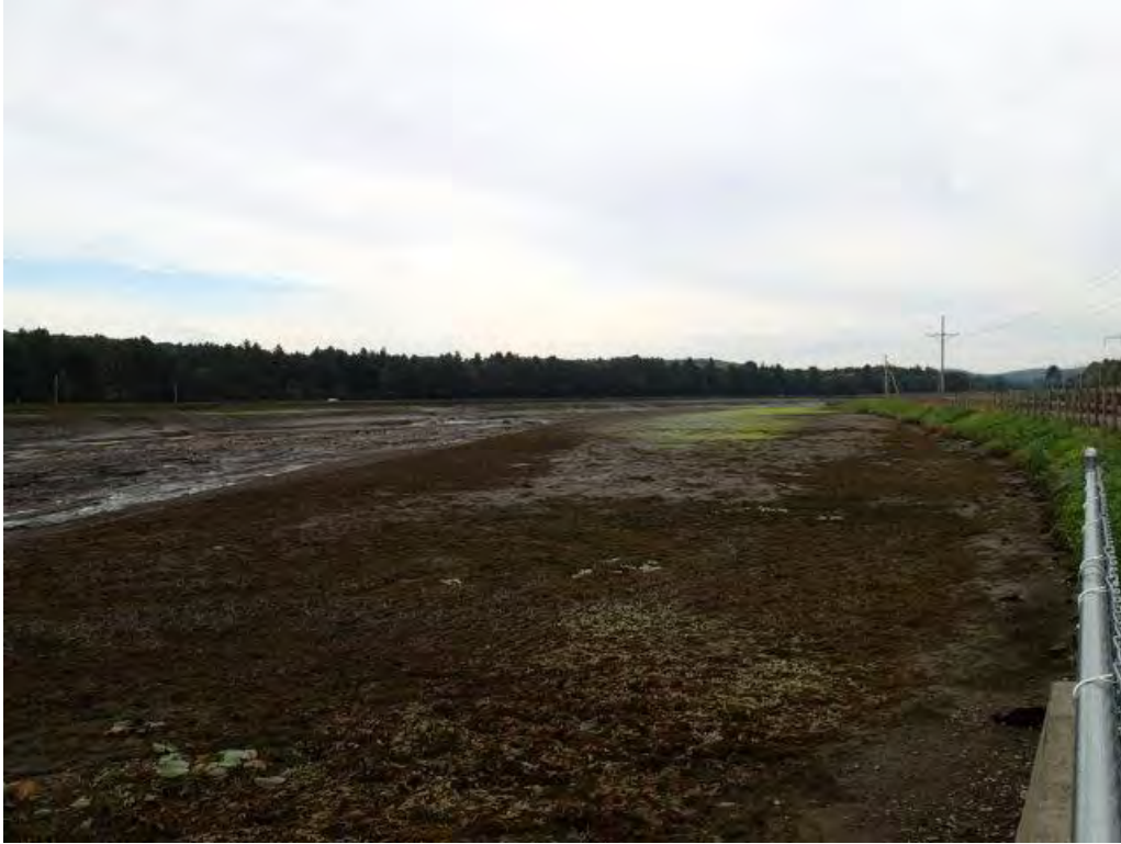
Photo 5. View from left bank of Zone 2 looking upstream (Day 1).
