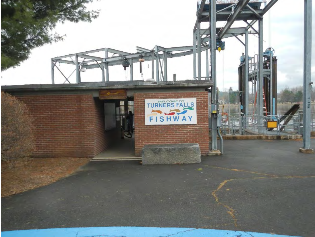
Figure 4.3-1 Fishway Viewing Facility Entrance
