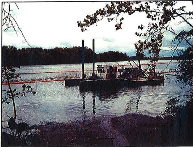
Northfield Mountain Dredging
