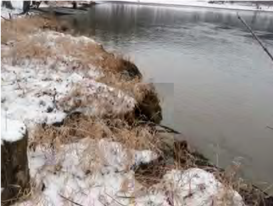
Photo No. 56 ( fluvial scouring along upstream end of island )
