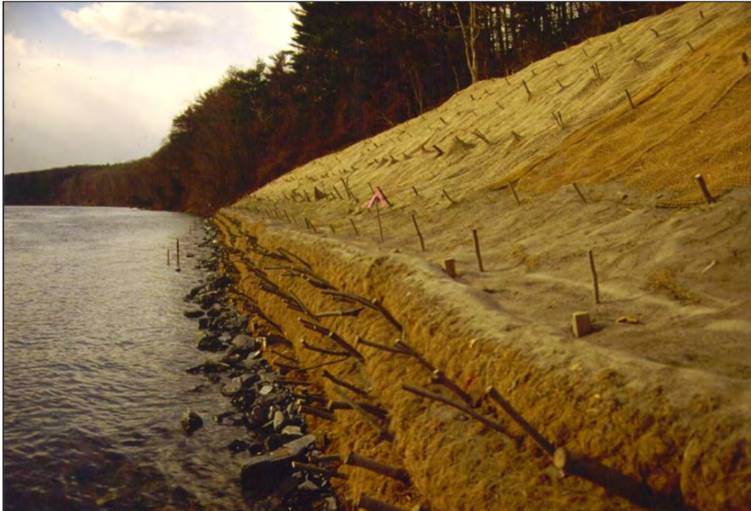
Photo 1: Wickey following construction, 1996
