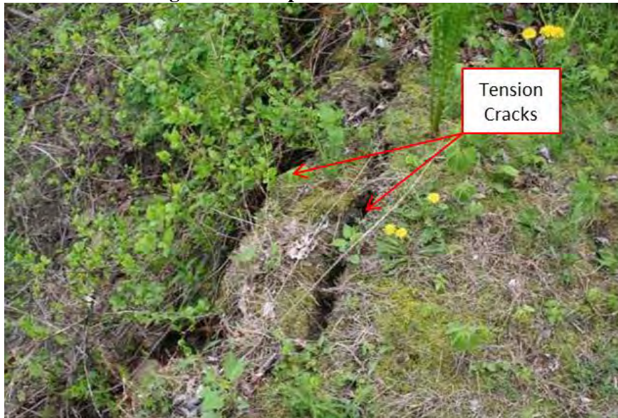
Figure 3: Example of Tension Cracks
