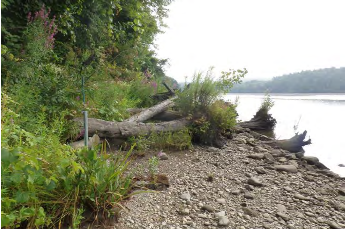
Figure 6.21 Vegetation planted on lower riverbank at stabilization site
