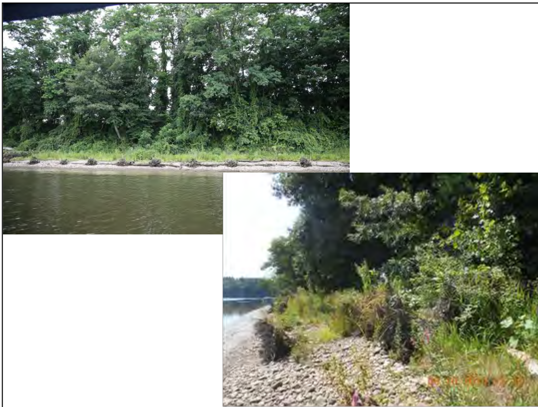
Photo 36: Upper Split River Farm I- Post Construction 2014. Detail from August, 2014
