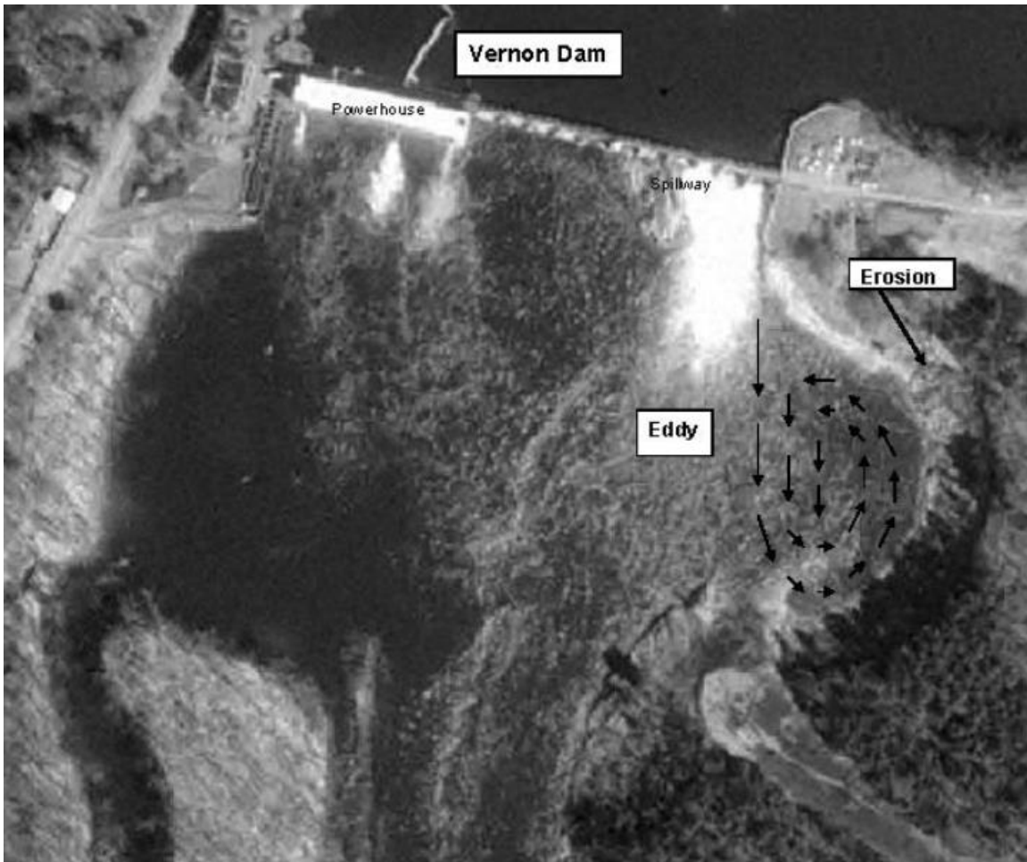
Figure 6.27 Eddy-induced erosion at Vernon Dam
