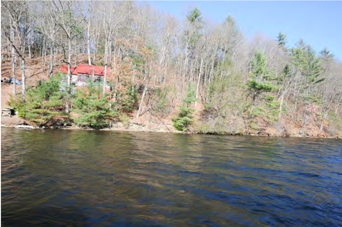
Figure 6.29 Erosion adjacent to seasonal Camp 2-W
