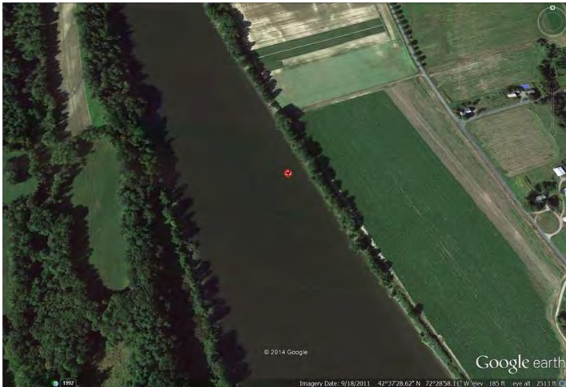
Figure 6.31 Aerial view of eroded riverbank adjacent to agricultural land-use
