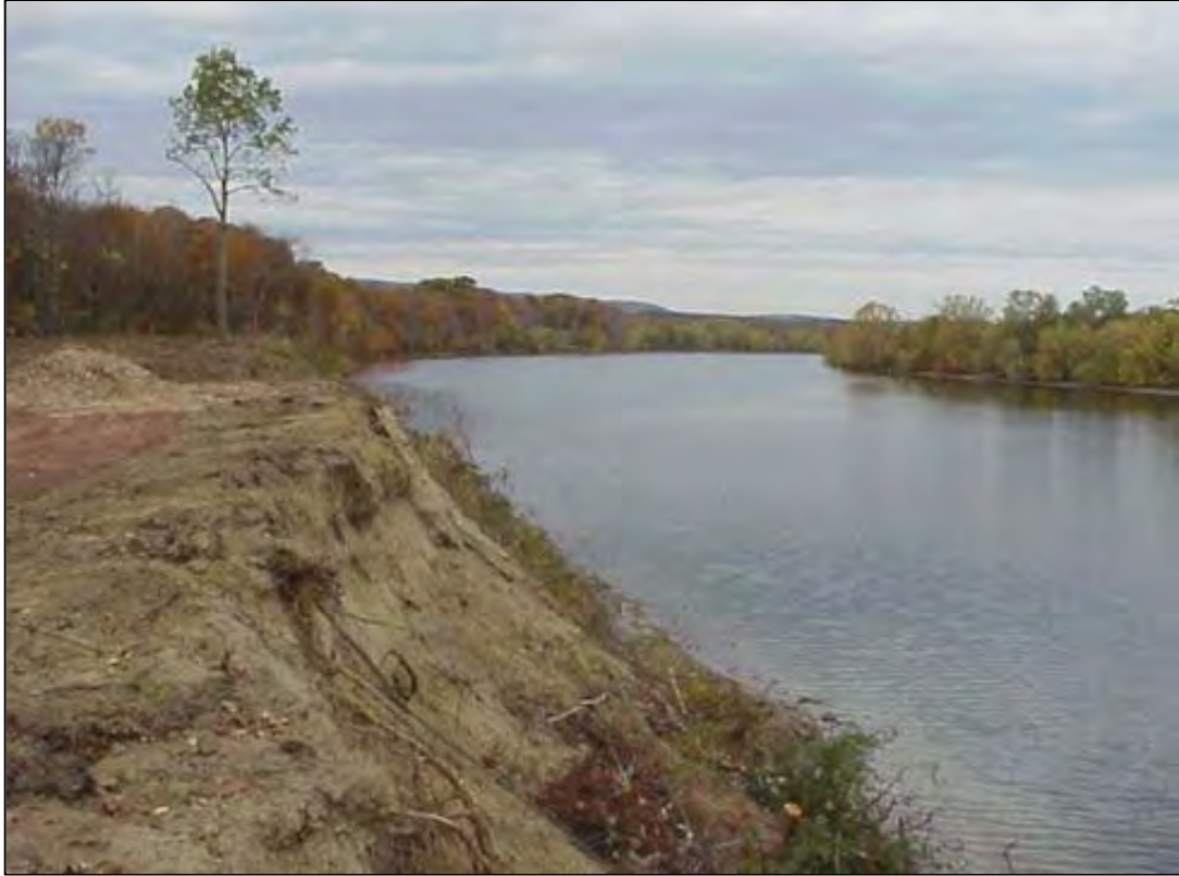
Photo 11: Urgiel Upstream pre- construction, 2001
