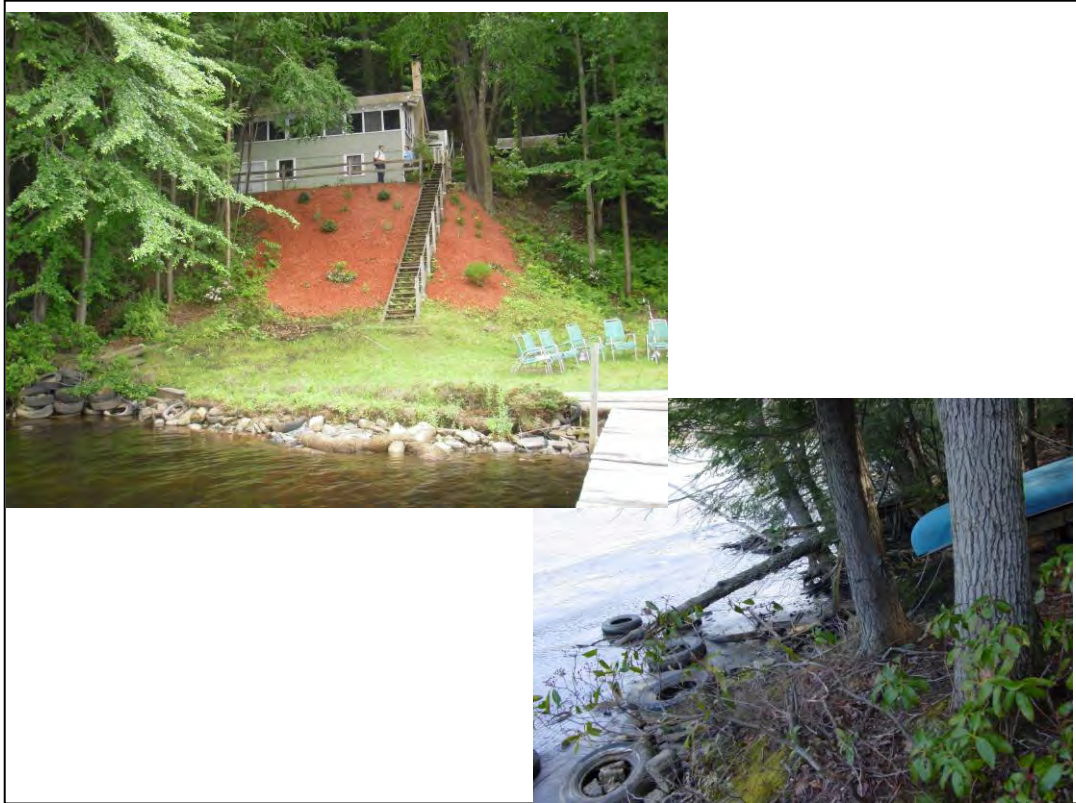
Photo 49: Camp 8E pre-construction 2011. Detail of bank
