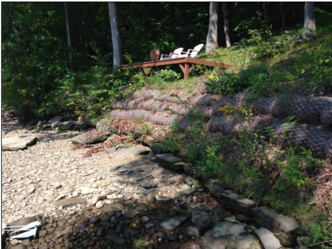
Photo 42: Camp 2W Post Construction 2014.
