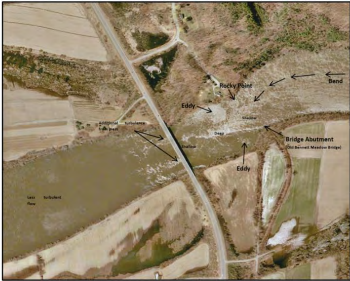
Figure 6.28 Eddy-induced erosion at Route 10 Bridge
