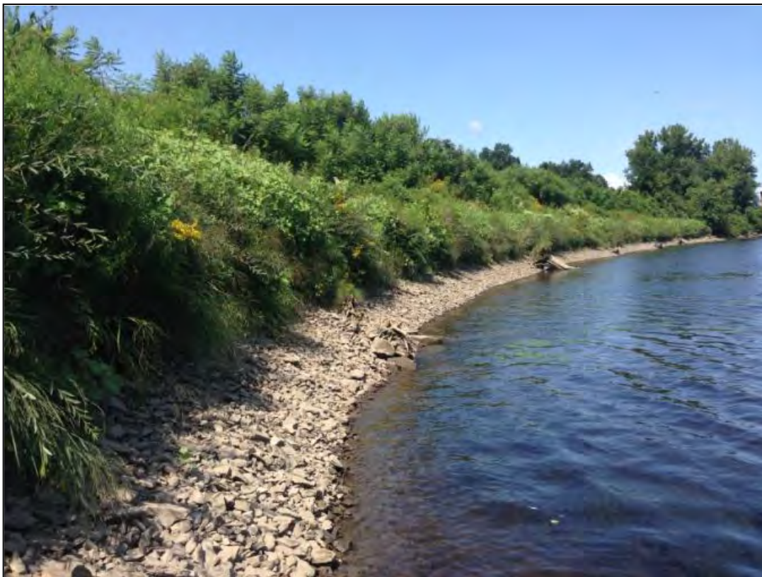
Photo 32: Kendall Farm- Post Construction 2014
