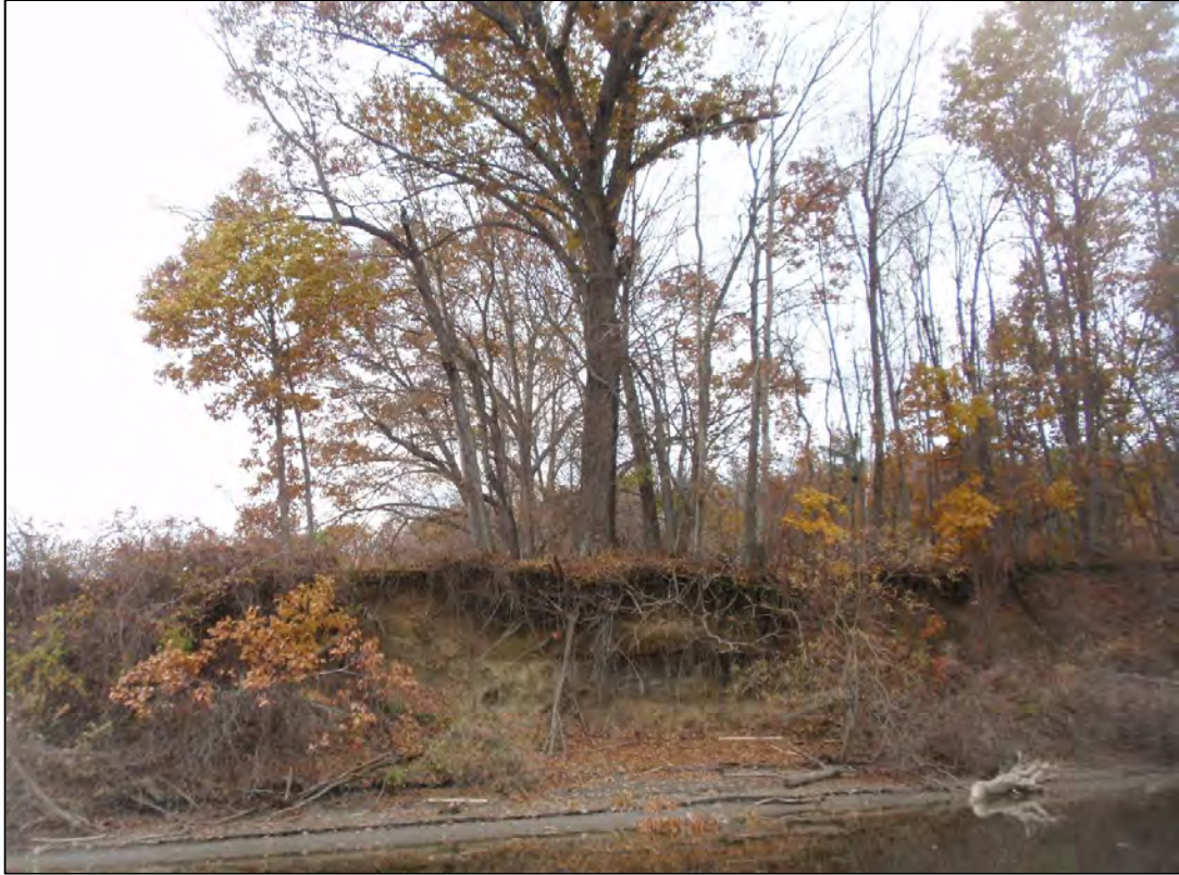
Photo 39: Bathory/Gallagher & Wallace/Watson pre-construction 2012
