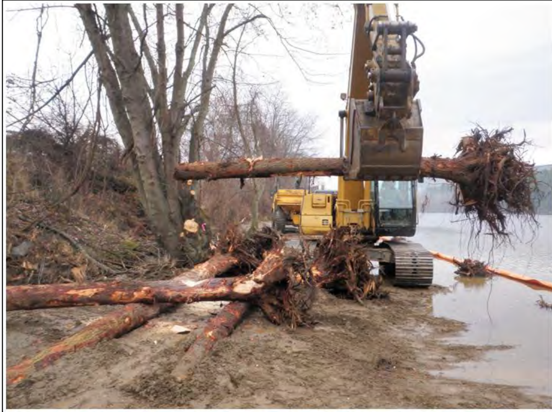
Photo 33: Lower Split River Farm- construction 2009
