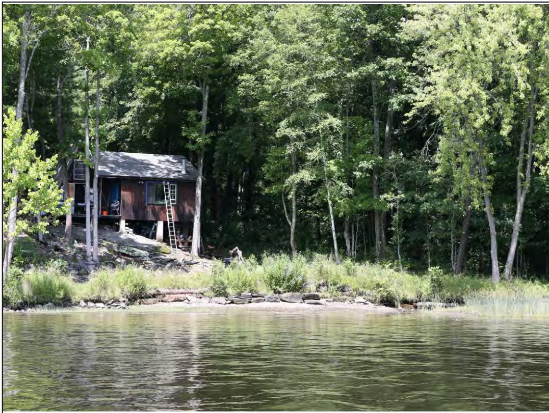
Photo 52: Camp 10W Post Construction 2014.
