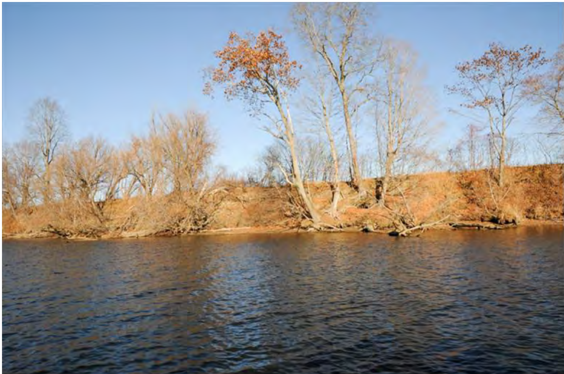
Figure 6.20 Eroded site (Segment 90), 2013
