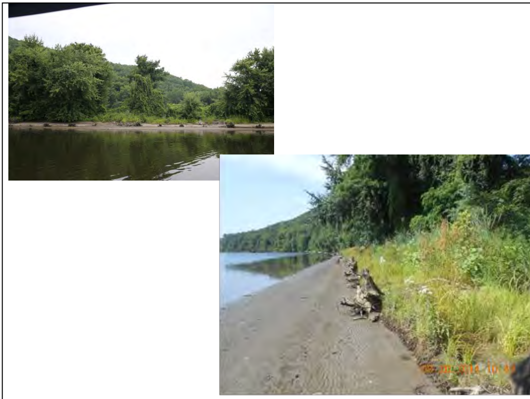
Photo 34: Lower Split River Farm- Post Construction 2014. Bank Detail from August, 2014
