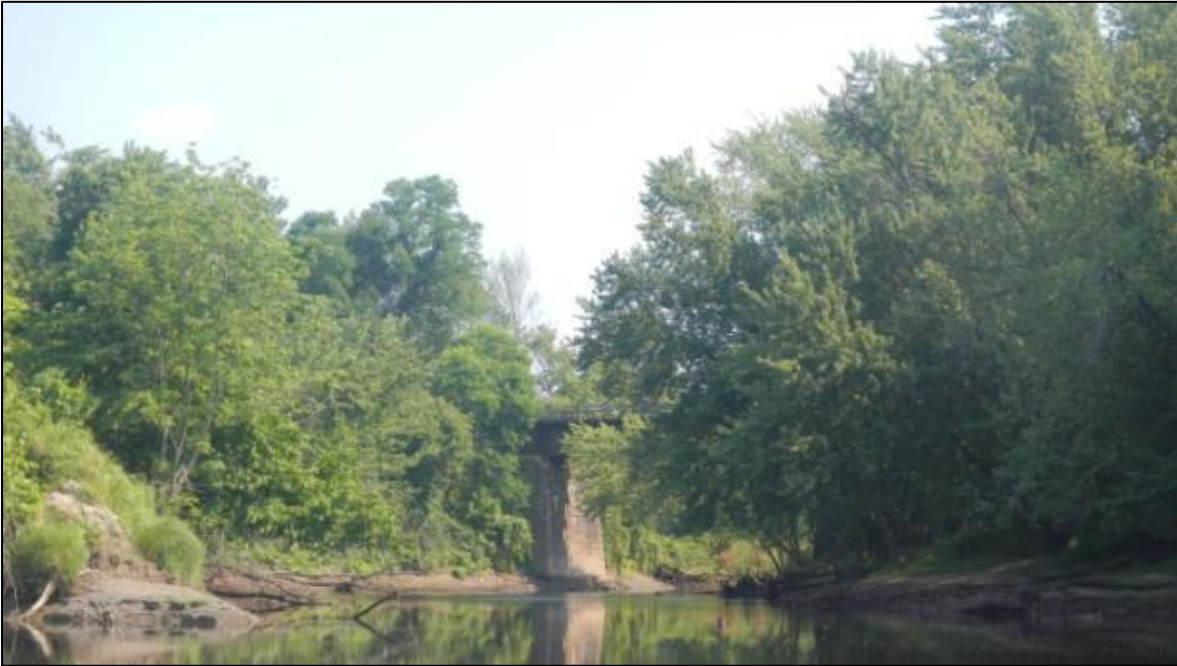
Ashuelot River Outlet to the Connecticut River
