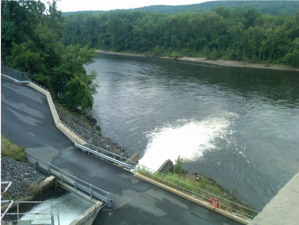
View of Sluice Gate discharge (approximately 210 cfs) from top of downstream fishway
