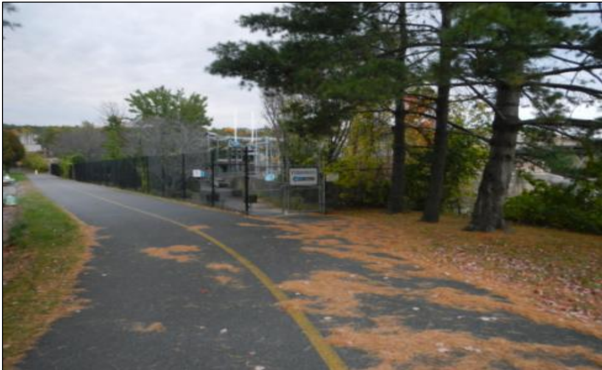
Access for the Fishway Viewing Area
