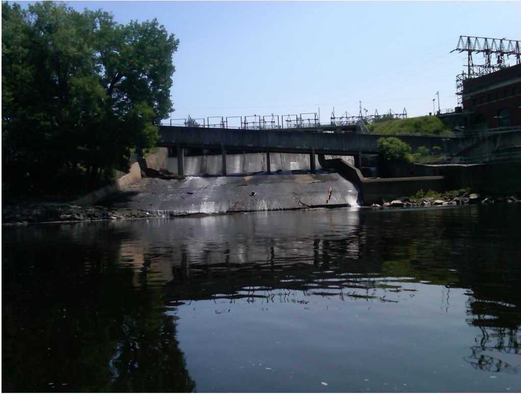
Upstream View of Spill Gate discharge location (no spill)
