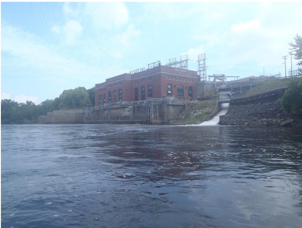
Upstream View of Sluice Gate discharge location
