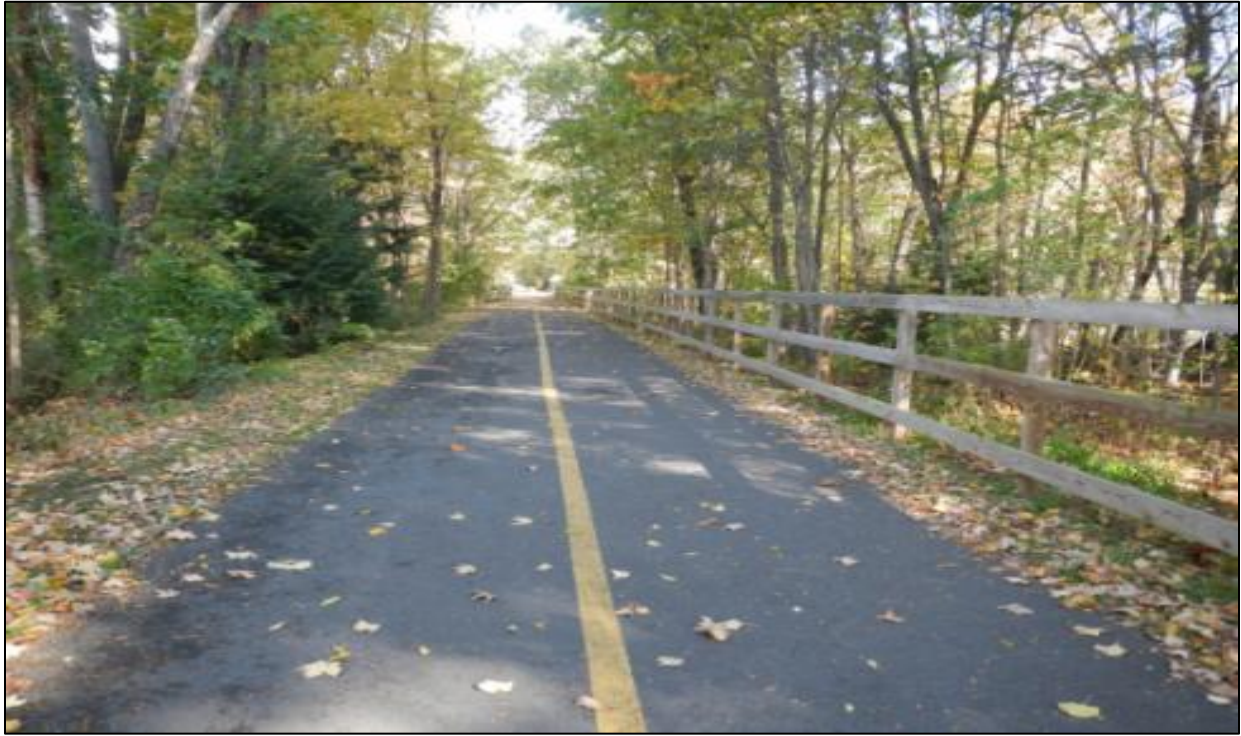
Typical Photo of Bike Trail
