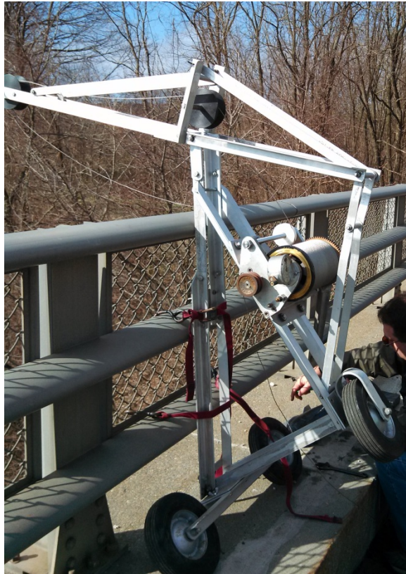
Crane and reel used to suspend LISST-100X from Route 10 Bridge
