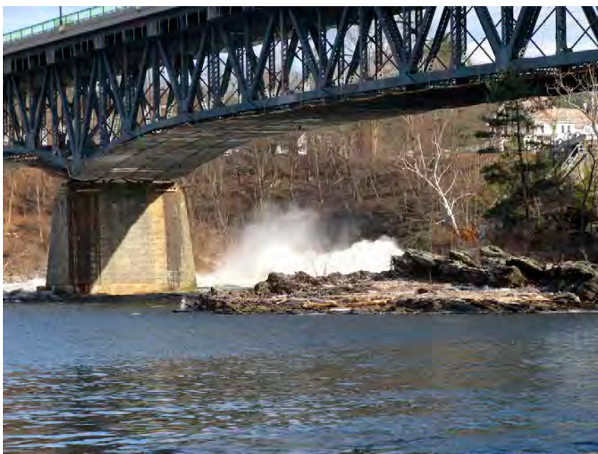
Turners Falls bypass reach with low flow, Feb. 1, 2013
