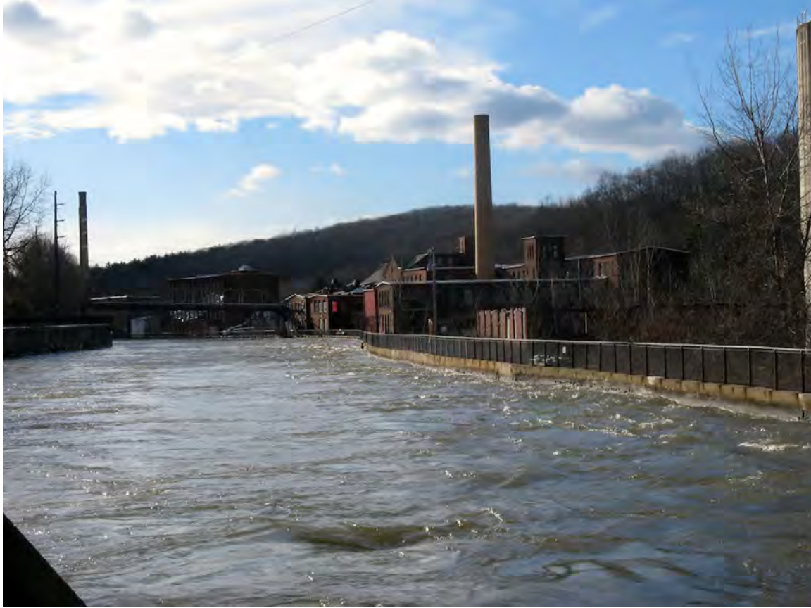
Turners Falls diversion canal.
