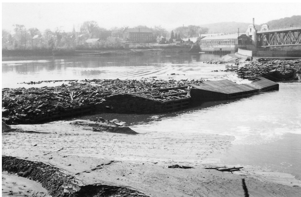
Remnants of the 1865 timber-crib dam were revealed during construction in 1969-71. (Photo courtesy Ed Gregory archive.)
