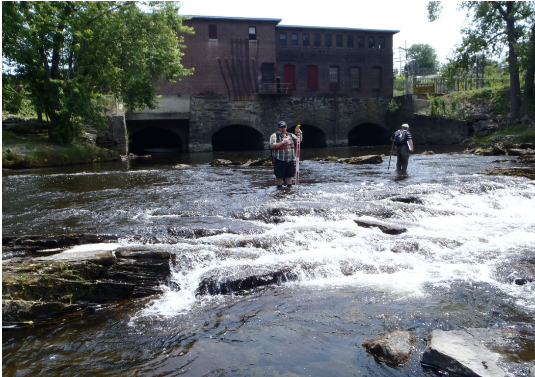
Figure 2.1.5b – View of Station No. 1 from Bypass Channel
