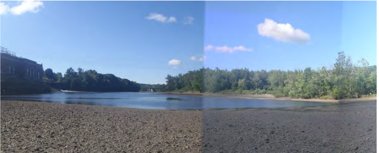
PHOTO 16. View looking downstream at confluence of backwater with Cabot Station tailrace
