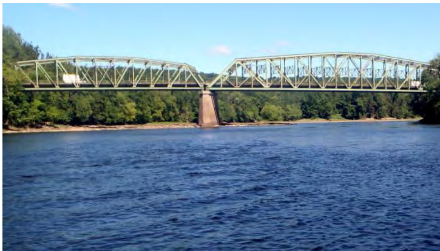
Photo 20. View looking upstream from pool toward ledge hydraulic control from Photo 17 ( exposed ledge can be seen under left chord of the General Pierce Bridge )
